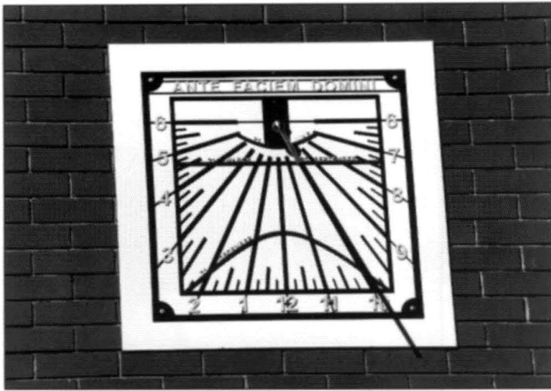
Figure 1. Time and date sundial for Christian Brothers College, Adelaide, South Australia, 1200x1200x3 mm stainless steel, powder coated.
